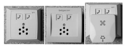
The VDSL modem shall be connected to the left RJ jack OR to the RJ11 jack of the 6 pins plug, with an appropriate patch cord.
